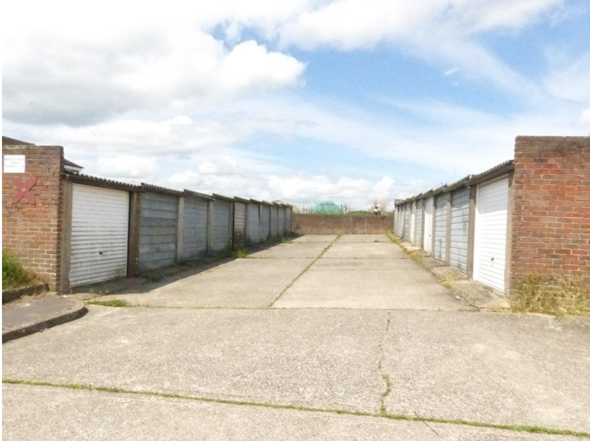
Martlett Road Garages 1-23
